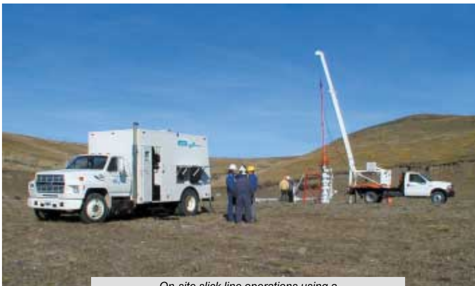
On-site slick line operations using a Ford 700 Slick Line Truck and F4000 Crane and Pick-up
