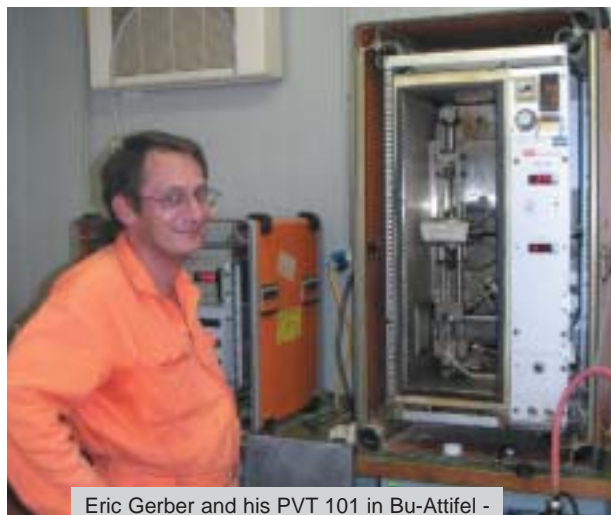
Eric Gerber and his PVT 101 in Bu-Attifel - still going strong after ten years of service
