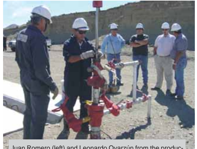
Juan Romero (left) and Leonardo Oyarzún from the production assistance team being observed changing the packing on a "Nodding Donkey" by, from right to left: Alfredo Valles (Supervisor), Sebastian Jelusic (IRAM Auditor), Tito Haro (Supervisor) and Pedro Yapura (Supervisor).
